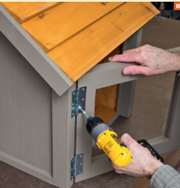
11. Add the door glazing and reinstall the door after finishing the structure.
