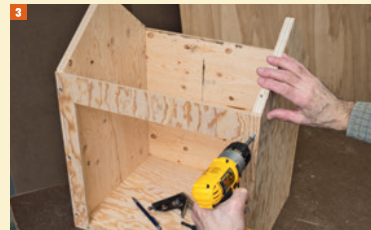
1. The bevel on the roof deck will span about half the thickness of the plywood. 2. Drill a starter hole at each corner, then make the door cutout with a jigsaw. Be sure to cut the narrow sides first. 3. The front and back panels fit over the sides, and all vertical pieces fit over the base.
